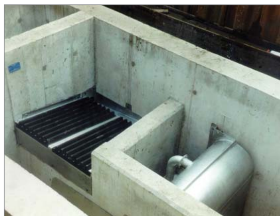
The Hydro-Jet® Screen differs from conventional screening systems because the flow is passed across the surface of the screen rather than perpendicular to the screen.
