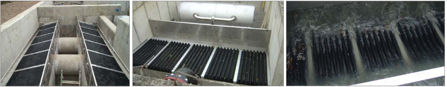
Continuous backwashing action cleans debris from screens.
